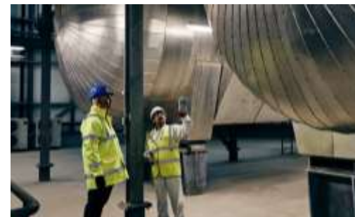
2024 Energy from waste, recycling & marine logistics
